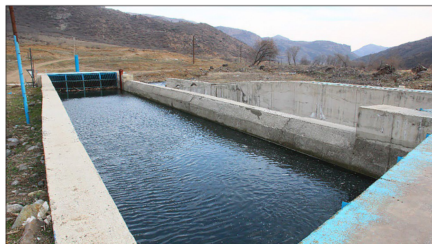
Figure 2. Rectangular sedimentation tank with 1 chamber
