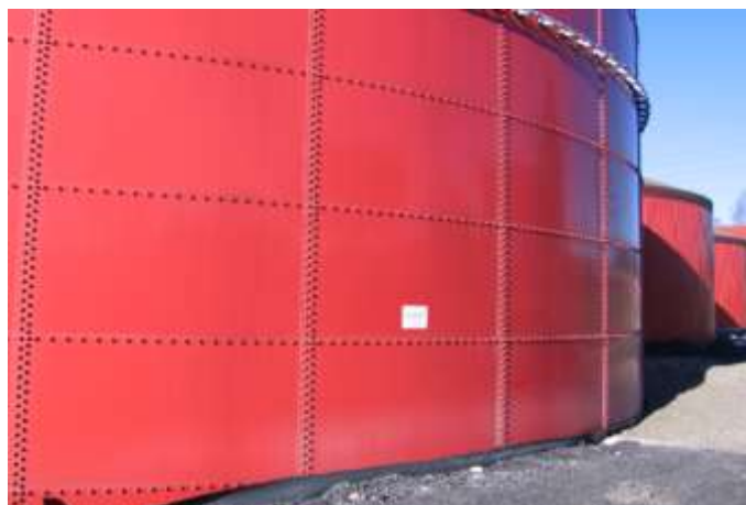
Fig. 5. Fermenters made of enamel metal sheets (photo J. Cebula)
