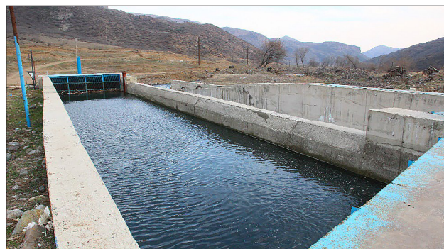
Figure 2. Rectangular sedimentation tank with 1 chamber
